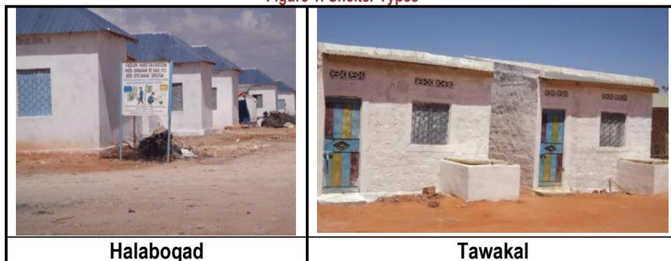
Throughout the planned settlements two main shelter designs were observed: cement block and CGI shelters. NRC provided 533 concrete hollow block houses in Halaboqad; 471 concrete homes were also built by UN-Habitat in Tawakal. In line with the less-secure land tenure situation at Salama One, DRC oversaw the construction of 250 corrugated-iron shelters there.
