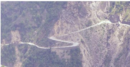
**Picture 3: Rockfall blocking access to the road to Lamabagar.**
